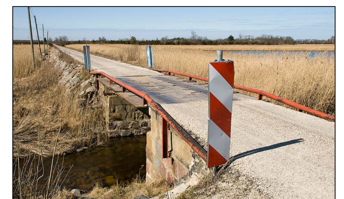
Endisel raudteetammil on nüüd autotee. Now there is a road on the previous railroad dam
